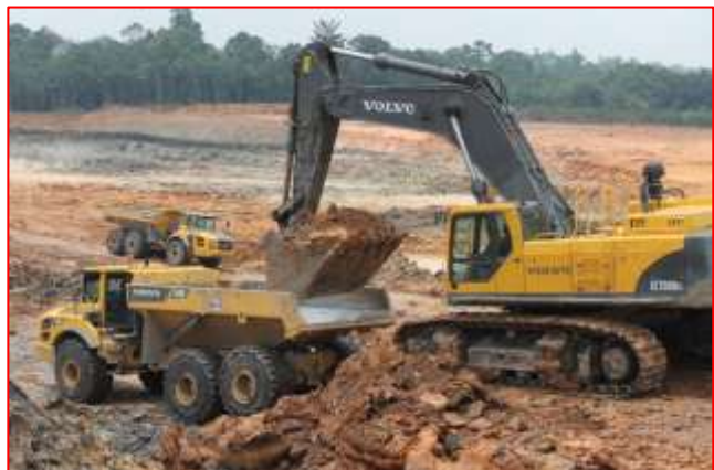
SEM Coal Mine: Pit 2 (Back fill in progress)
