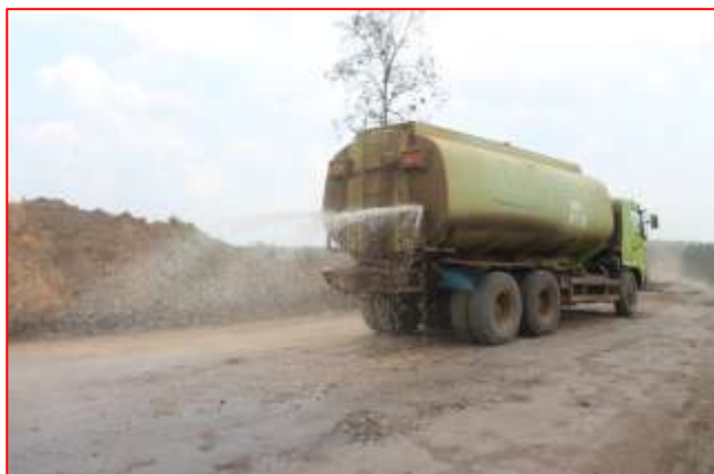
Regular road maintenance and widening
