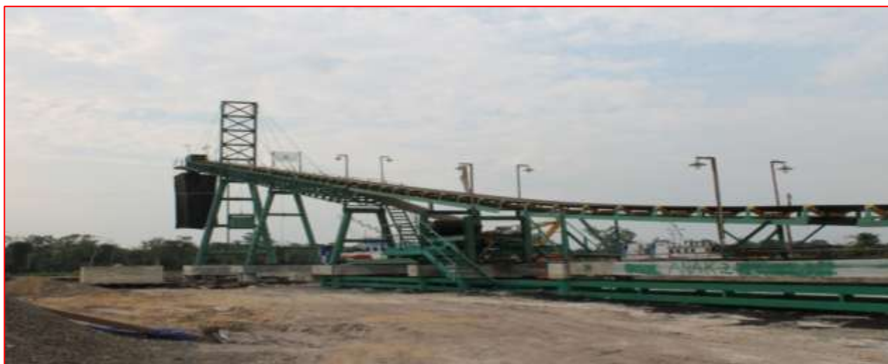
Conveyor belt at jetty
